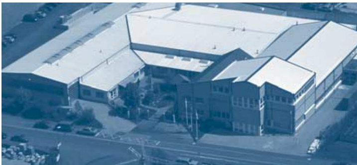
Cassel Messtechnik GmbH (Germany) – Headquarters and main production site
